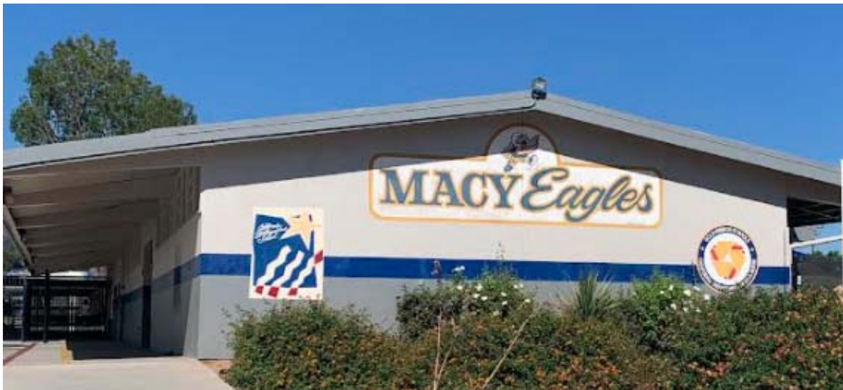
Macy ES: Roofing, HVAC, Fire Alarm, Sewer, Storm Drain
