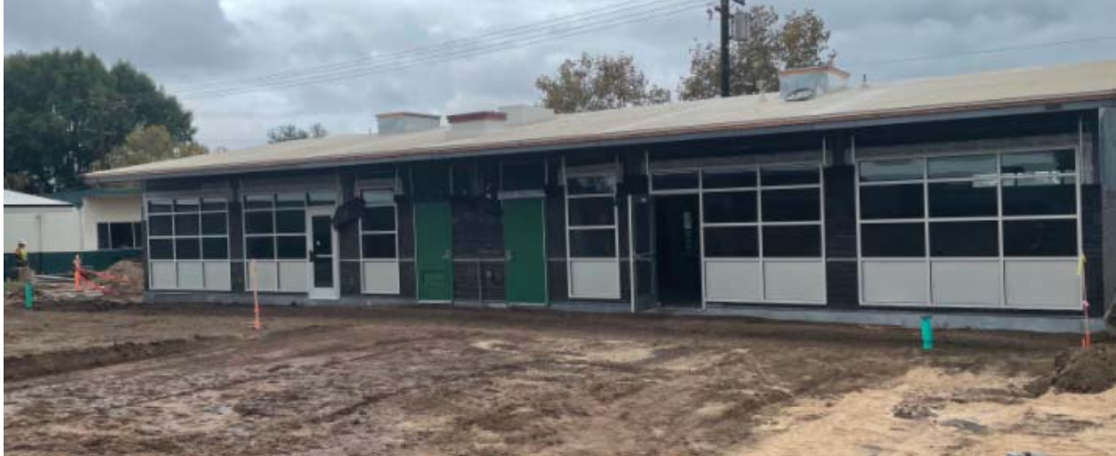
Jordan ES: Roofing, HVAC, Fire Alarm, Sewer, Portable to Permanent
