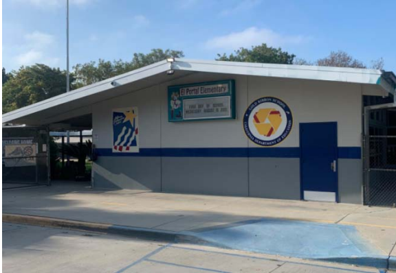
El Portal ES: Roofing and Fire Alarm
