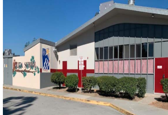
Olita ES: Roofing, HVAC, and Fire Alarm
