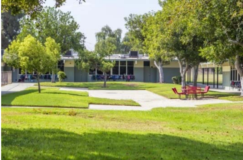
Meadow Green ES: Roofing, HVAC, Fire Alarm, Sewer
