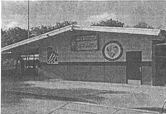
El Portal ES: Roofing and Fire Alarm
