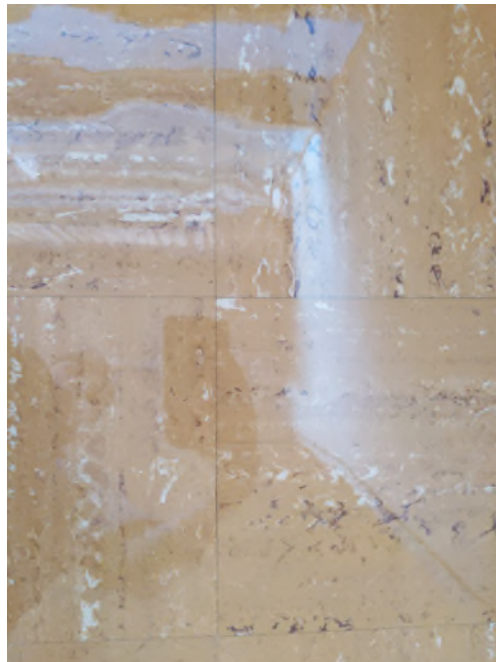
View of 9"x 9" Orange/Brown Resilient Flooring/Resilient Floor Mastic
