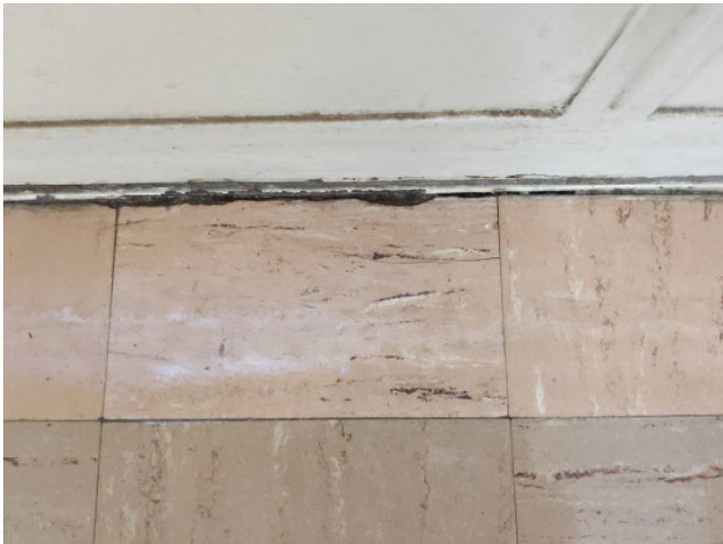
View of 9" x 9" Red/Brown Streaked Resilient Flooring/Resilient Floor Mastic
