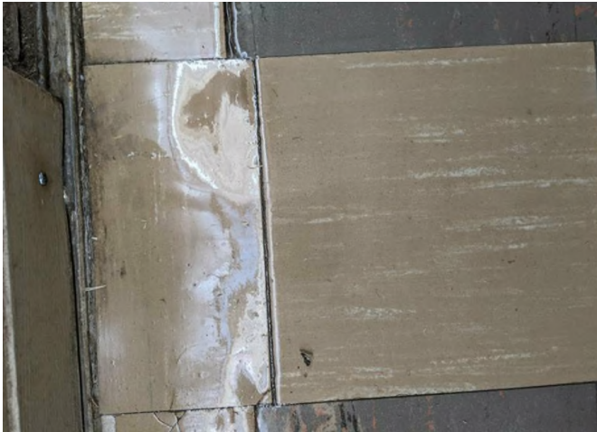
View of 9"x9" Light Brown with Tan Streaked Resilient Flooring/Resilient Floor Mastic
