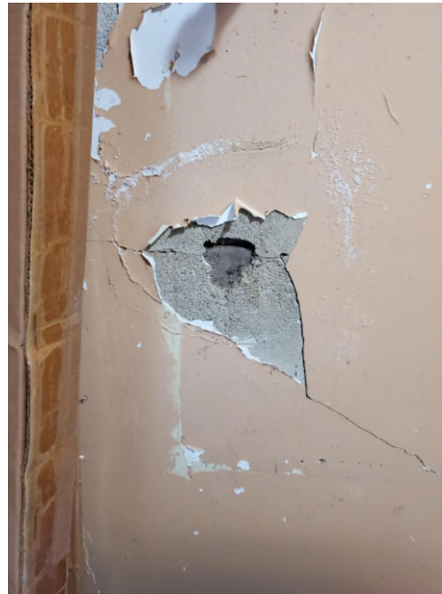
View of Plaster on Buttonboard
