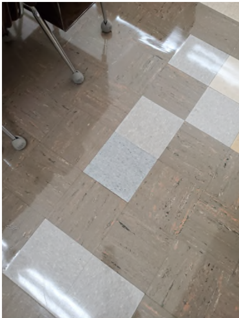
View of 9" x 9" Gray Speckledd Resilient Flooring/Resilient Floor Mastic
