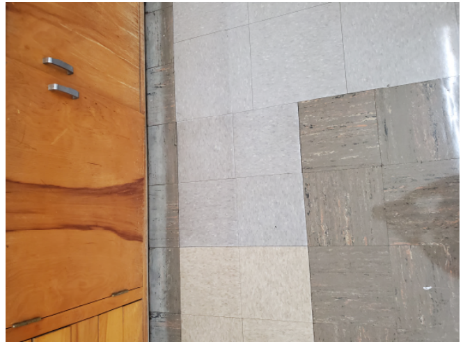
View of 9"x 9" Gray with White Streaked Resilient Flooring/Resilient Floor Mastic
