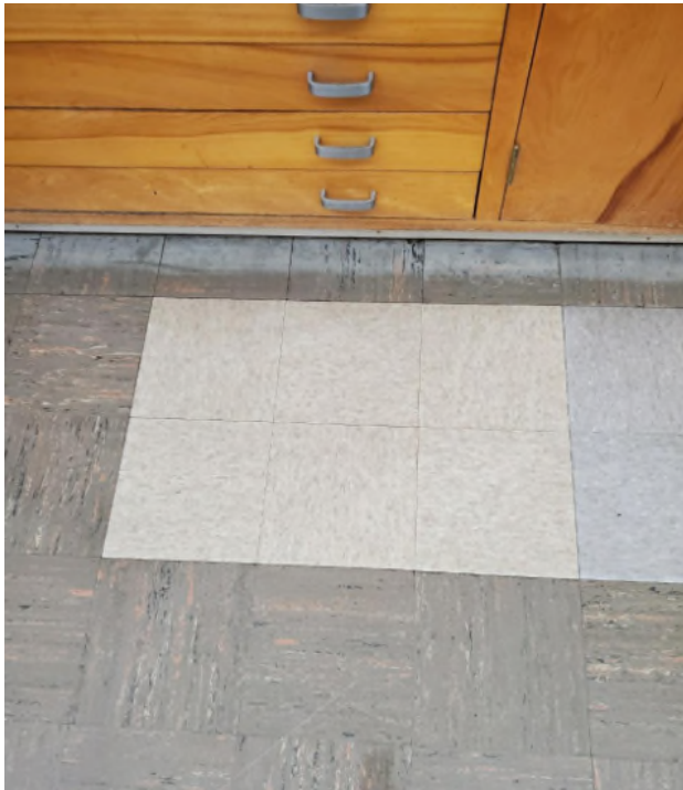
View of 9"x9" Tan Speckled Resilient Flooring/Resilient Floor Mastic
