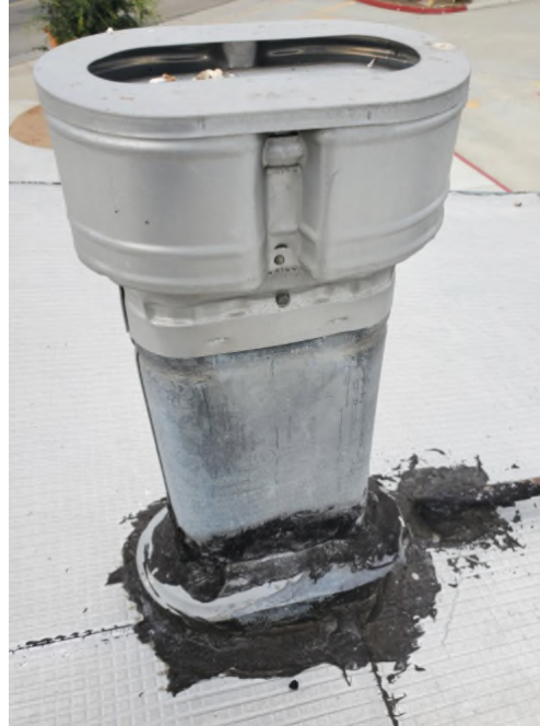
View of Black Roof Penetration Mastic
