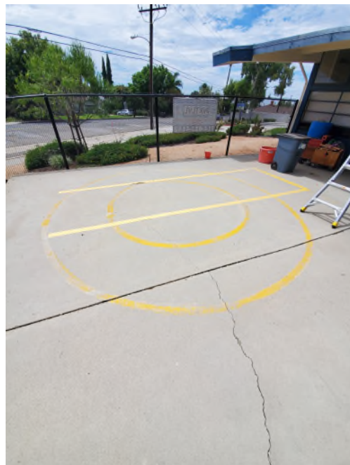
View of Yellow Concrete Floor
