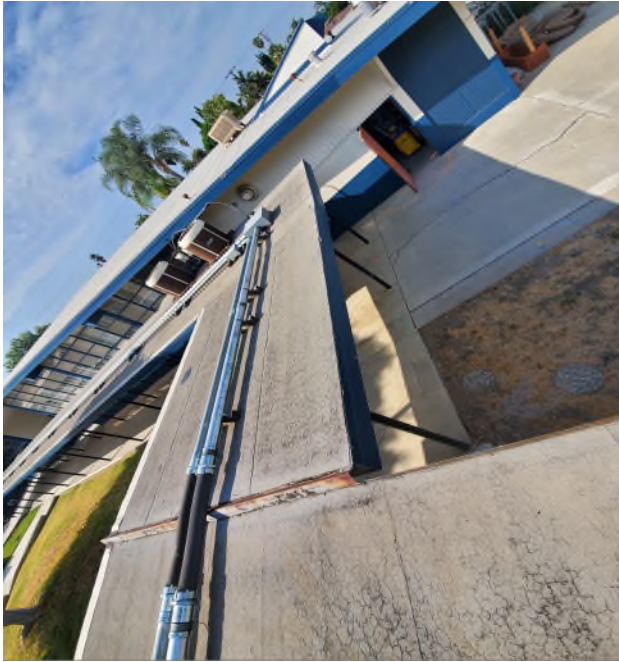
View of Blue Metal Flashing
