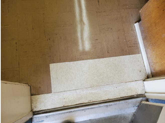
View of 9"x9" White Speckled Resilient Flooring/Resilient Floor Mastic
