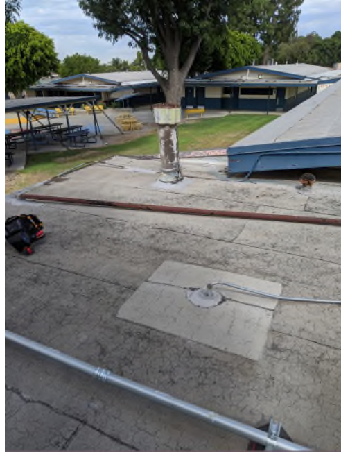
View of 9" Diameter Transite Pipe
