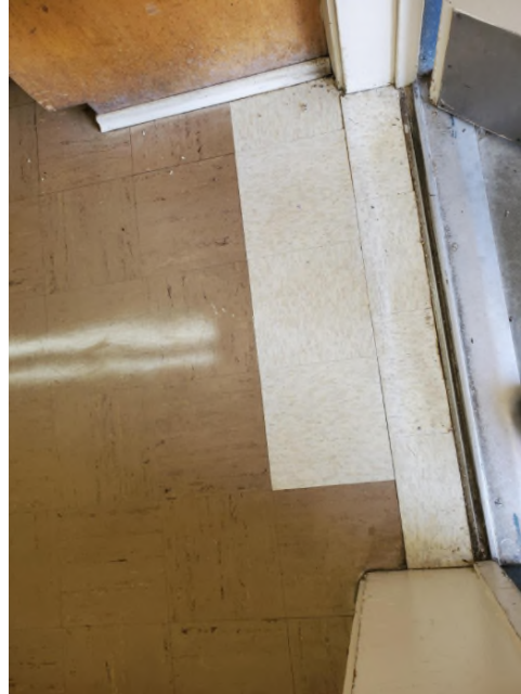
View of 9"x9" Dark Tan Resilient Flooring/Resilient Floor Mastic
