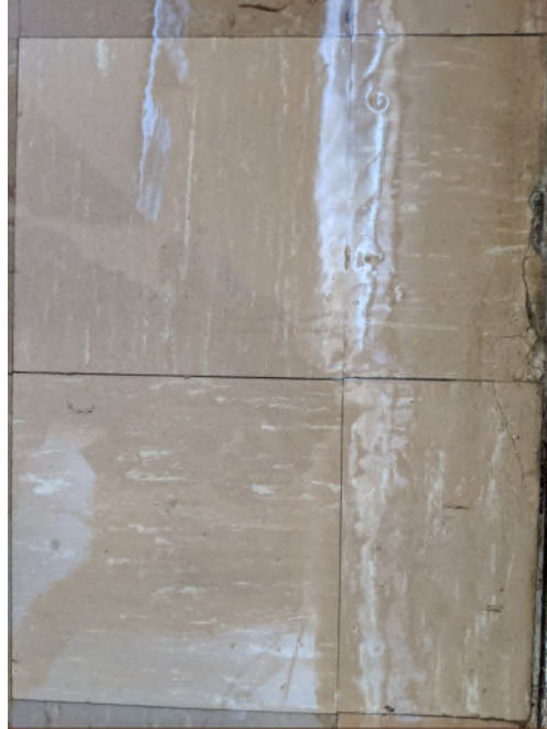
View of 9"x 9" Gray Streaked Resilient Flooring/Resilient Floor Mastic
