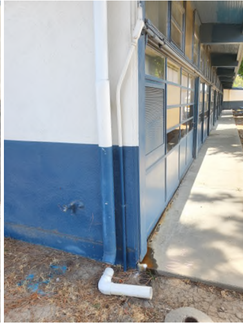
View of Blue Metal Rain Gutter
