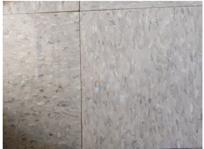
View of 9"x 9" Blue/Gray Streaked Resilient Flooring/Resilient Floor Mastic
