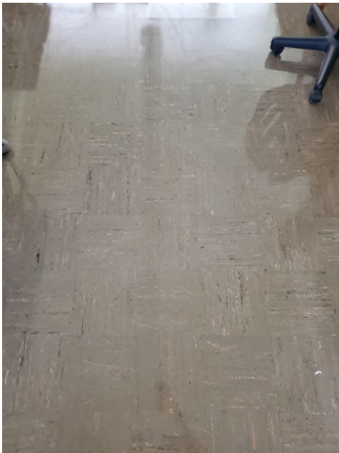
View of 9"x 9" Dark Gray with Pink Streaked Resilient Flooring/Resilient Floor Mastic
