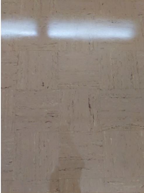
View of 9"x 9" Brown Streaked Resilient Flooring/Resilient Floor Mastic
