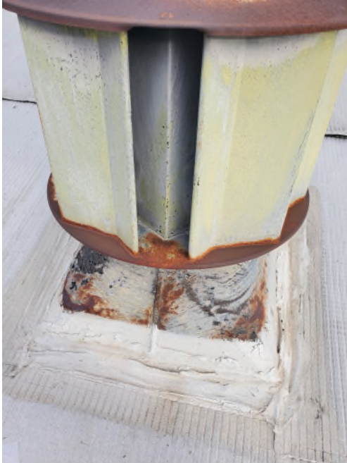
View of Gray & White Roof Penetration Mastic
